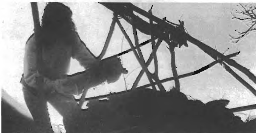
Geri places a flat rock on chimney as rain cap (above).
