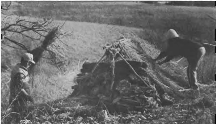
Long grasses are placed on the roof, overlapping the sides and several inches thick. Some pieces of bark are placed on the very peak to help this vulnerable area to shed water.
