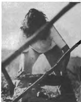
Geri places a flat rock on chimney as rain cap (above).
