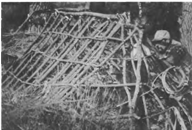
Lashing together the framework.
